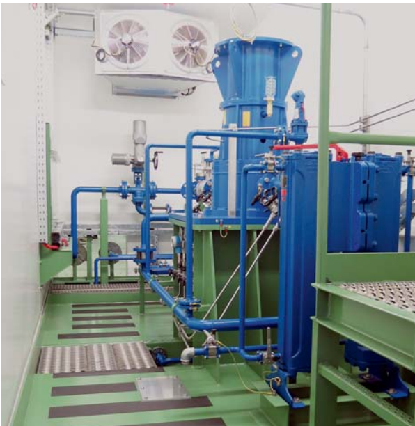
High-pressure pump skid with vertical double casing pump
