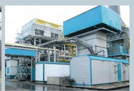
The Vyngapur gas processing plant (SiburTyumenGaz) processes associated petroleum gas from the Gazprom Neft fields into the dry stripped gas and a broad fraction of light hydrocarbons.
